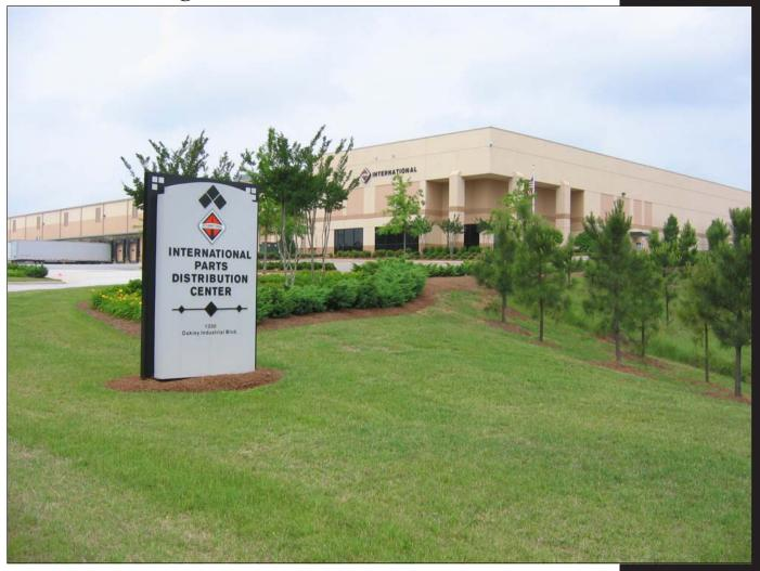
Navistar International Truck and Engine is a new 350,000 SF heavy equipment automotive facility located in Fairburn, Georgia. Construction of this project included load bearing concrete tilt-up panels with interior structural steel columns, a steel frame roof structure, heavy duty reinforced floor slabs, and ESFR sprinkler systems. The facility also includes 3,000 SF of office space, and high pile storage in racks. RACO was awarded the contract as Design-Build Prime Contractor.
