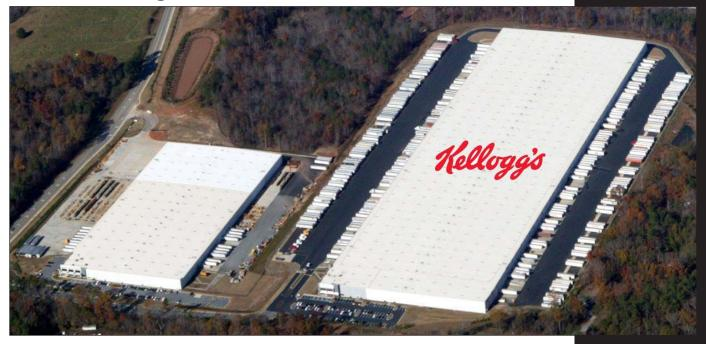
The Kelloggs Distribution Center is a new 903,000 SF food grade distribution plant located in Atlanta, Georgia. Construction of this project included load bearing concrete tilt-up panels with interior structural steel columns, a steel frame roof structure, heavy duty reinforced floor slabs, and ESFR sprinkler systems. The facility also includes 18,000 SF of office space and high pile storage in racks. RACO was awarded the contract as Design-Build Prime Contractor.
