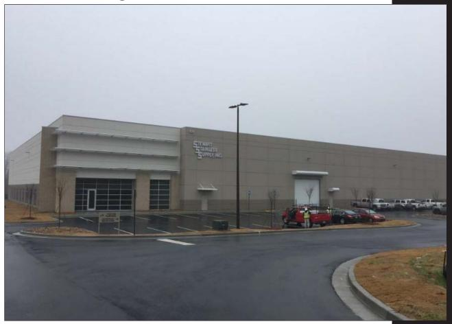
Stewart Stainless Supply is a 130,000 SF stainless steel light fabrication and machining/distribution center located in Braselton, Georgia. Construction of this project included load bearing concrete tilt-up panels with interior structural steel columns, a steel frame roof structure, heavy duty reinforced floor slabs, and machine foundations. The facility also included 10,000 SF of office space. RACO was awarded the contract as Design-Build Prime Contractor.
