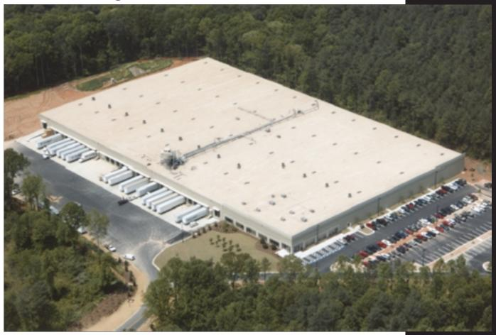
RACO has completed numerous projects for the retail display manufacturer including three distribution/manufacturing facilities in Acworth. Construction of these projects included load bearing concrete tilt-up panels with interior structural steel columns, a steel frame roof structure, heavy duty reinforced floor slabs, and ESFR sprinkler systems. The facilities total over 539,000 SF and also include over 20,000 SF office space. RACO was awarded these contracts as Design-Build Prime Contractor.
