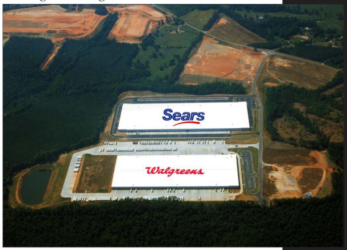
Jackson 85 Distribution and Warehouse facilities are located in Pendergrass, Georgia. Construction of these projects include load bearing concrete tilt-up panels with interior structural steel columns, a steel frame roof structure, heavy duty reinforced floor slabs, and ESFR sprinkler systems. RACO was awarded the contract Design-Build Prime Contractor.
