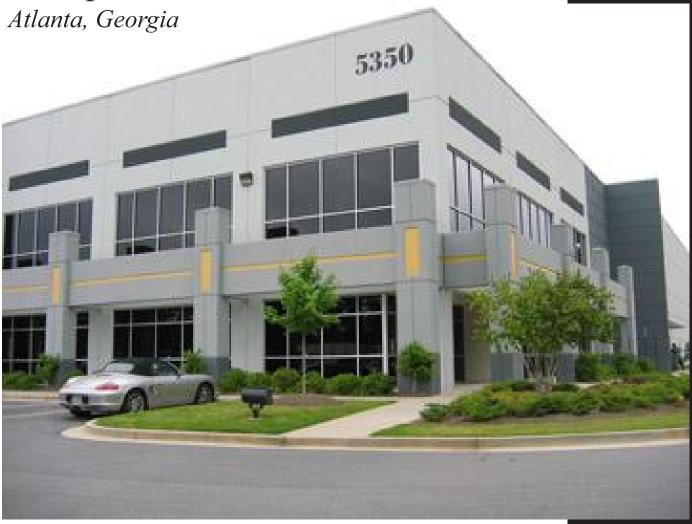
Caterpillar, Inc. is a new 220,000 SF heavy equipment manufacturing facility located in Atlanta, Georgia. Construction of this project included load bearing concrete tilt-up panels with interior structural steel columns, a steel frame roof structure, heavy duty reinforced floor slabs, and ESFR sprinkler systems. The facility also includes 10,000 SF of office space and high pile storage
