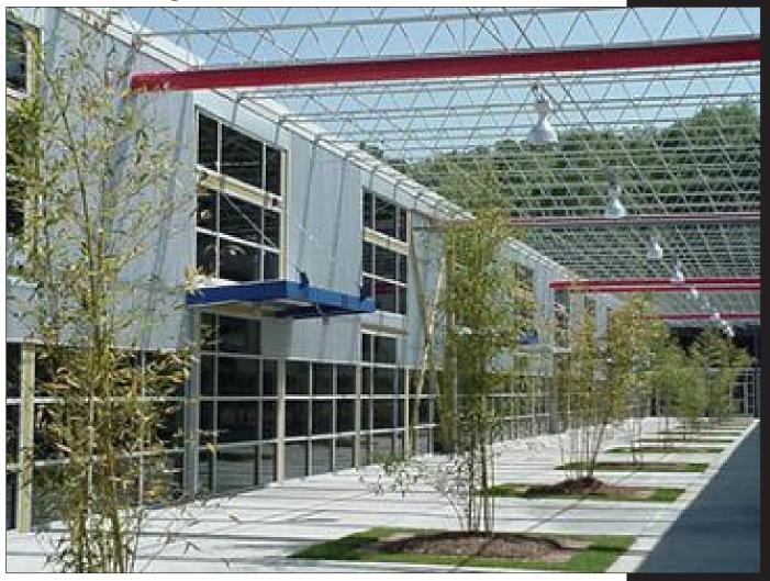
The Glassworks is a 45,000 SF office / condominium renovation in Atlanta, Georgia. Construction of this project was part of the urban renewal program, and included free standing steel panels, as well as veneer metal and masonry exterior walls. The facility also includes Class A office space. RACO was awarded the contract as Design-Build Prime Contractor.
